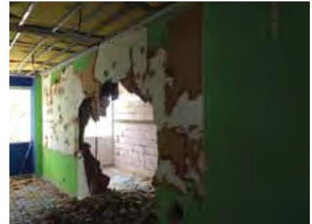
Need for space: four new rooms were created in the school building during the summer holidays (July 2014). This involved breaking down and building new walls, setting doors, installation of electricity and sinks, renewing the tiles, and adding new air conditioning units.
